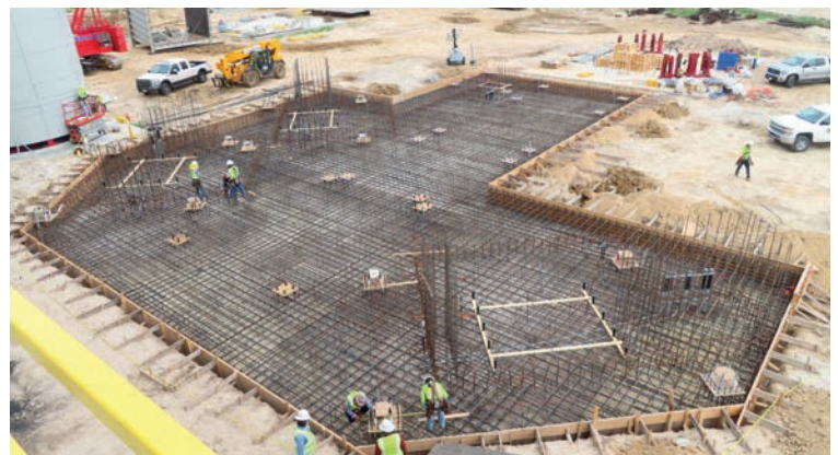
Above image shows the foundation for one of the baghouse outlets within the Steel Dynamics, Inc. construction projects. The image on page 2 shows the scale of the reverse air baghouses.
