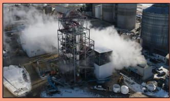
Adelphi Construction LC recently supplied structural steel and staircases for this Ethanol Plant project, plus provided specialty construction trade services to install a ring dryer and other process equipment including vertical centrifuges, horizonal decanters, pressure gravity screens, drag and screw conveyors, tanks, agitators, scrubber with internal packing, centrifugal pumps with seal pots, and a track operated building hoist. All work was performed during a time sensitive plant shutdown.
