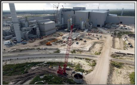
Steel Dynamics, Inc. (SDI), the greenfield EPC project in Sinton, TX, which includes two reverse air baghouses, pneumatic and mechanical conveying, storage silos, alloy additive systems, and more is nearing completion. Project Manage Will Michels said IAC and SDI teams are fully into the commissioning stage and working together to turn over the project completely to SDI.
