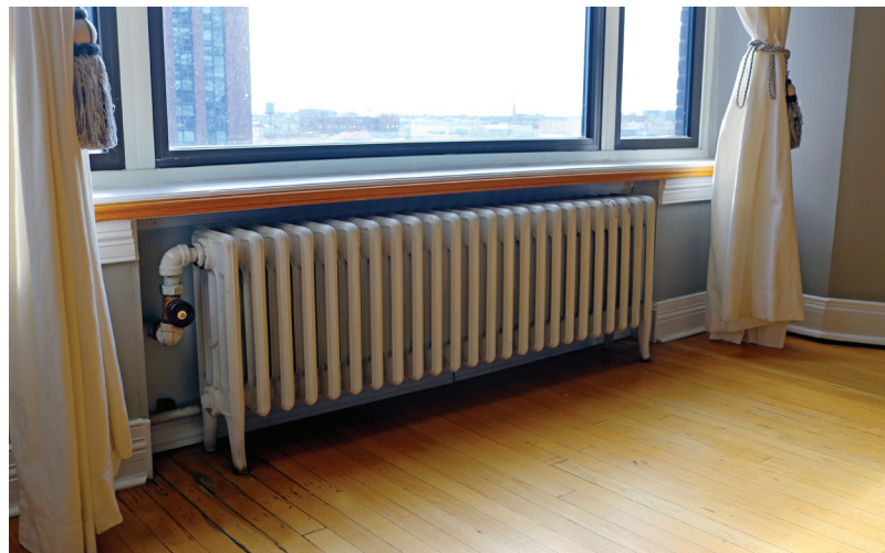
TESTED AND REPLACED STEAM TRAPS
