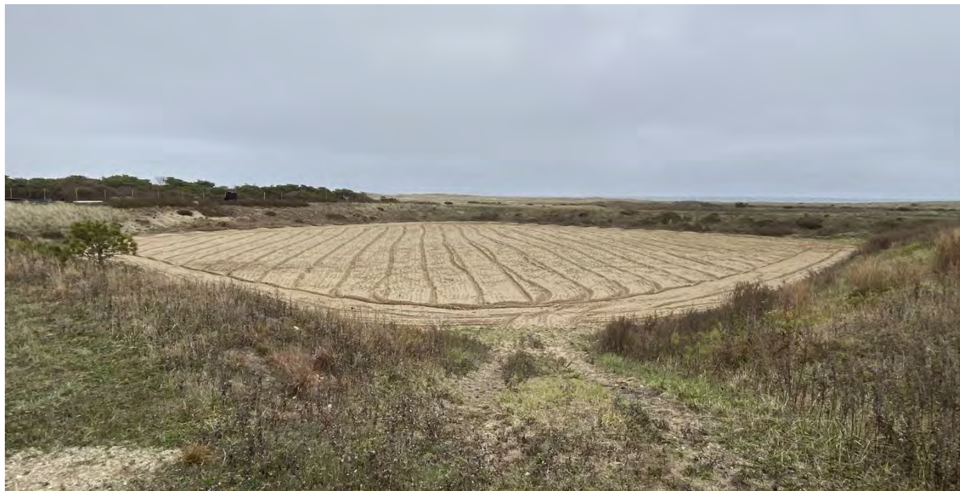
Settling Beds along coast at Surfside Waste Water Treatment Facility (photo by Chelsea Kilburn)
