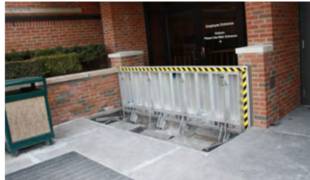
Top: Swing-hinged gate stored in recessed wall. PS Flood Barriers
