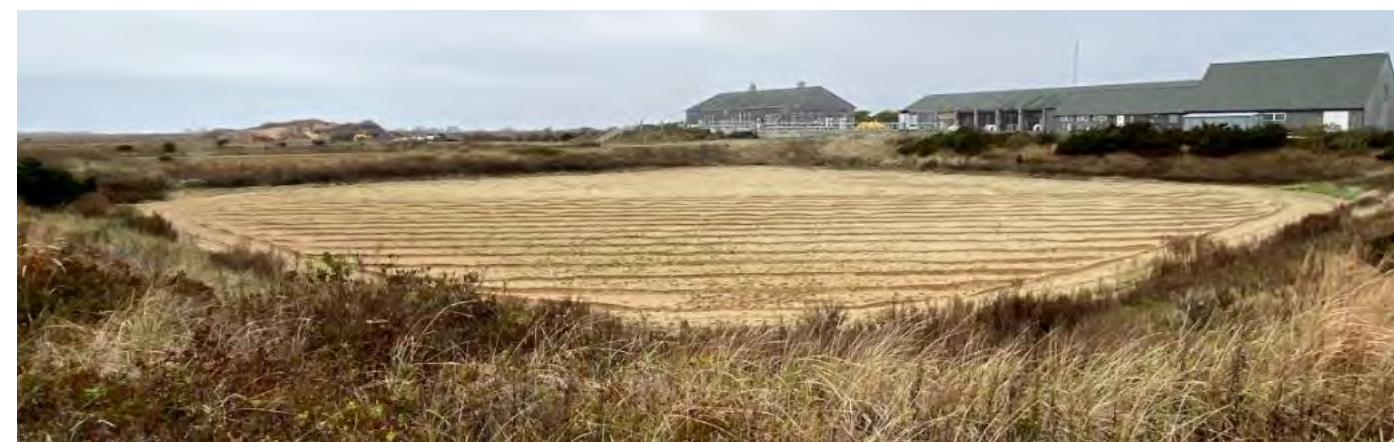
Wastewater Treatment Plant (photo by Chelsea Kilburn)
