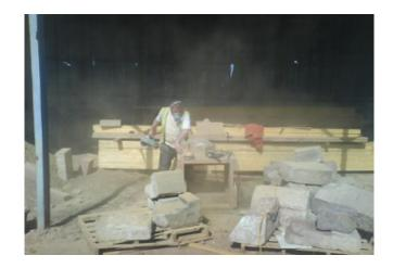
On site during the 1980s and 1990s power tools had become a necessity; their use increased production by 100 plus percent. The guys doing restoration works and repairs would spend days on end cutting into walls with angle grinders with no respiratory protection whatsoever. Most thought the clouds of dust they were producing were only a 'nuisance'.
