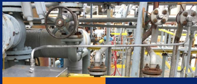
▲ The picture is a home made system and consists of a pipe from the process line to a sulfuric acid sample box. The pipe from the valve (top right) to the sample box (bottom left) must be purged before a representative sample can be taken. This not only produces waste, but if not flushed correctly leftover residue may influence the next sample.
