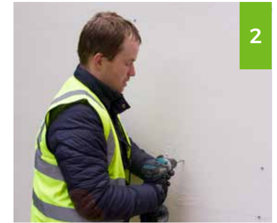
Drill the holes
