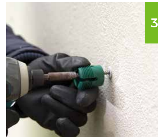
Plug & screw the fixing
