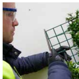
STEP 3 File the grid after cutting.
