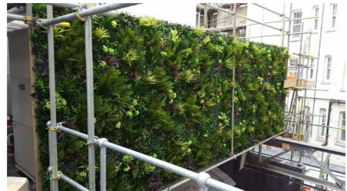
Completed project dressed with Delicate White Color Box prior to install due to complicated access to the wall
