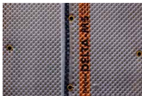
Delta Qwik-Seal Plug installed into the waterproof membrane
