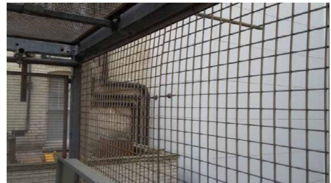
Metal cage before Signature Panel installation
