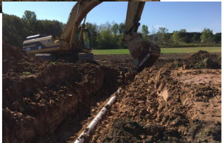
Photos of the wetland complex construction taken by Gary VanVreede on September 28, 2017. The photo above is site location #7 and the photo to the right is site location #1.
