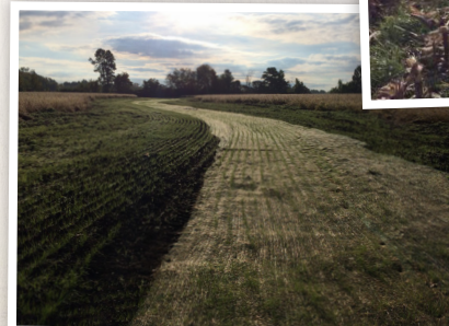
Grassed waterway installation
