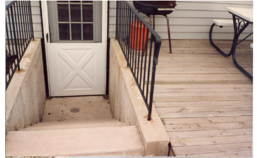
Stairwell with drain
