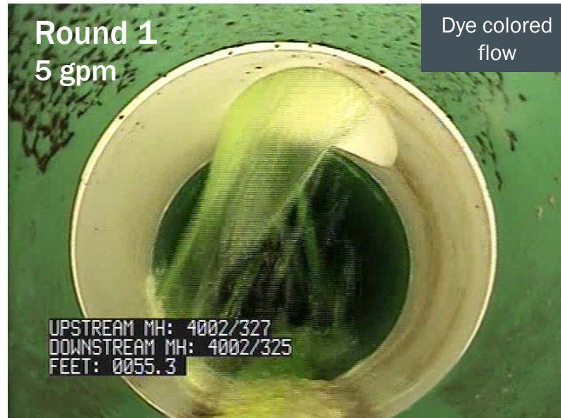
Round 1: New PVC sanitary main and lateral connector stub
