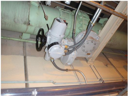
New Actuator for Air Valve AV-B5 in Tunnel
