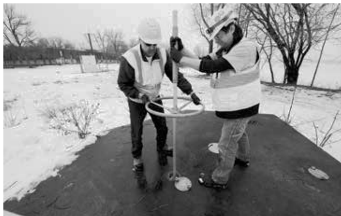
Field Services opening up a siphon barrel to allow more flow capacity to NEW Water's DePere facility
