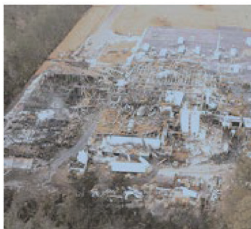
A pharmaceutical plant after a dust explosion.
