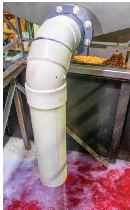
Screened wastewater is pumped to the municipal wastewater plant in compliance with accepted levels of total suspended solids.
