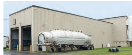
At the SBS Sparta facility, sugar is transferred from railcars to bulk trailers that carry the materials to their final destinations.
