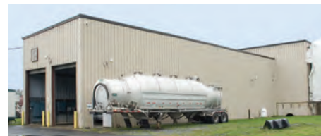
At the SBS Sparta facility, sugar is transferred from railcars to bulk trailers that carry the materials to their final destinations.
