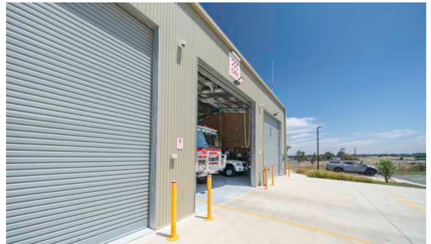
Locations / All emergency services buildings photography: Carlsruhe
