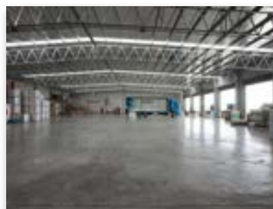
Open web truss
