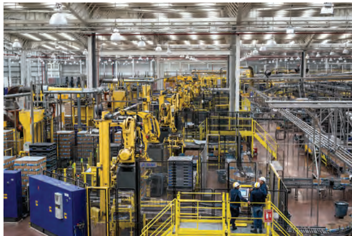
In just two years, Constellation Brands, Inc. expanded the existing capacity of its Nava Brewery in Mexico by 250 percent, making it the world’s largest brewery. The red outline marks the size of the original facility.
