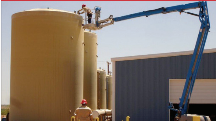
TANK BATTERY MAINTENANCE
