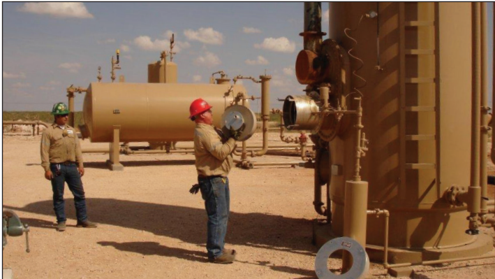
TANK BATTERY MAINTENANCE
