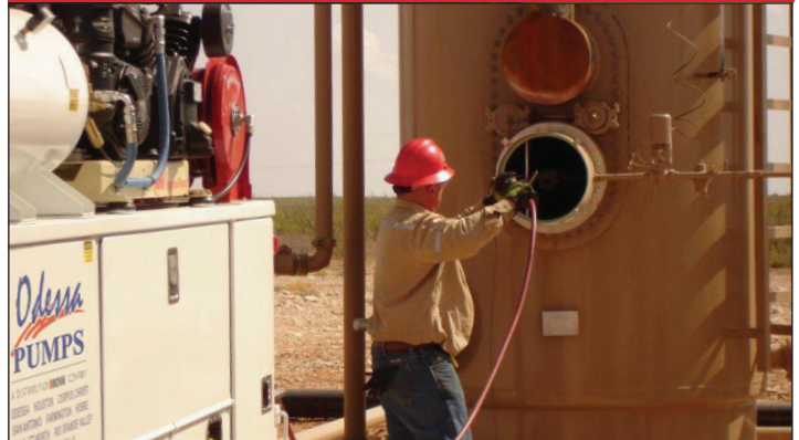
TANK BATTERY MAINTENANCE
