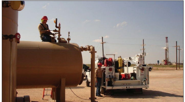
TANK BATTERY MAINTENANCE
