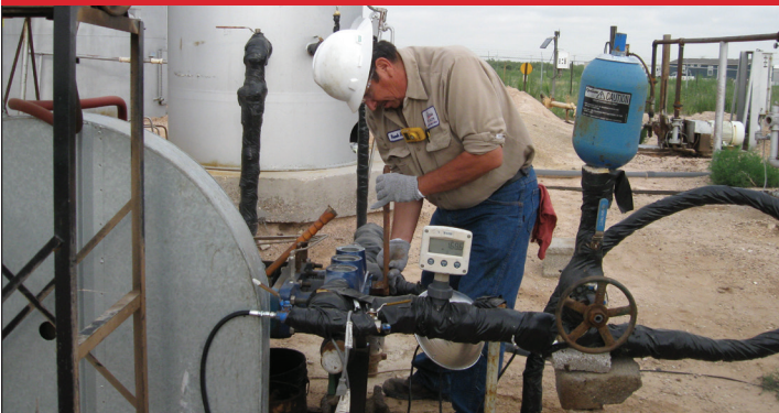
FIELD SERVICE REPAIRS
