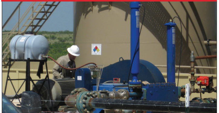
FIELD SERVICE START-UP
