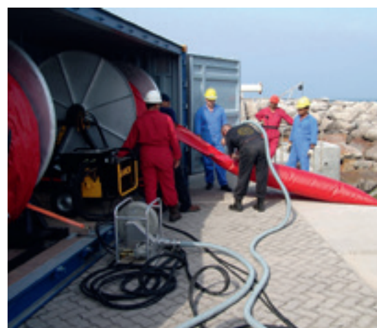
Inflatable Light Boom (PVC/PU & Neoprene), height: 650-1650 mm (26-65 in)
