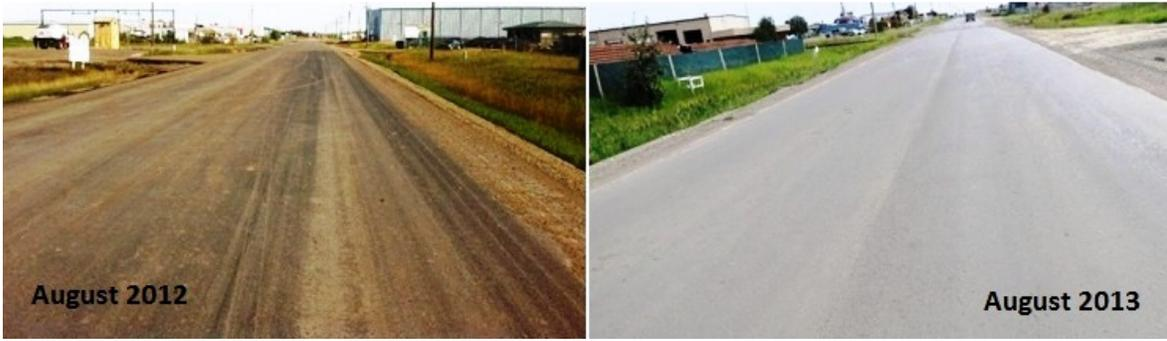
Figure 5: Paved road surface on NPA geocell-reinforced base (August 2012 and August 2013)
