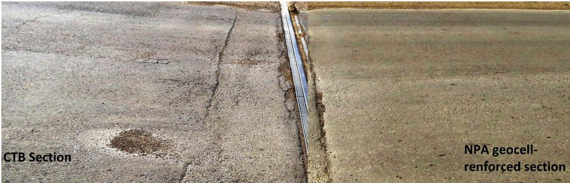
Figure 6: CTB section on left and NPA Geocell-reinforced on right side of rail track (Picture taken on August 2013)
