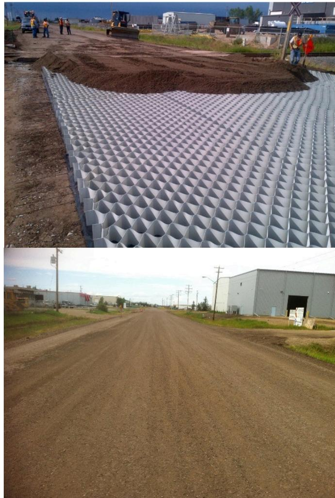
Figure 4: Fully stretched NPA geocell (top) and compacted NPA geocell-reinforced base (bottom) (picture taken in July 2012)
