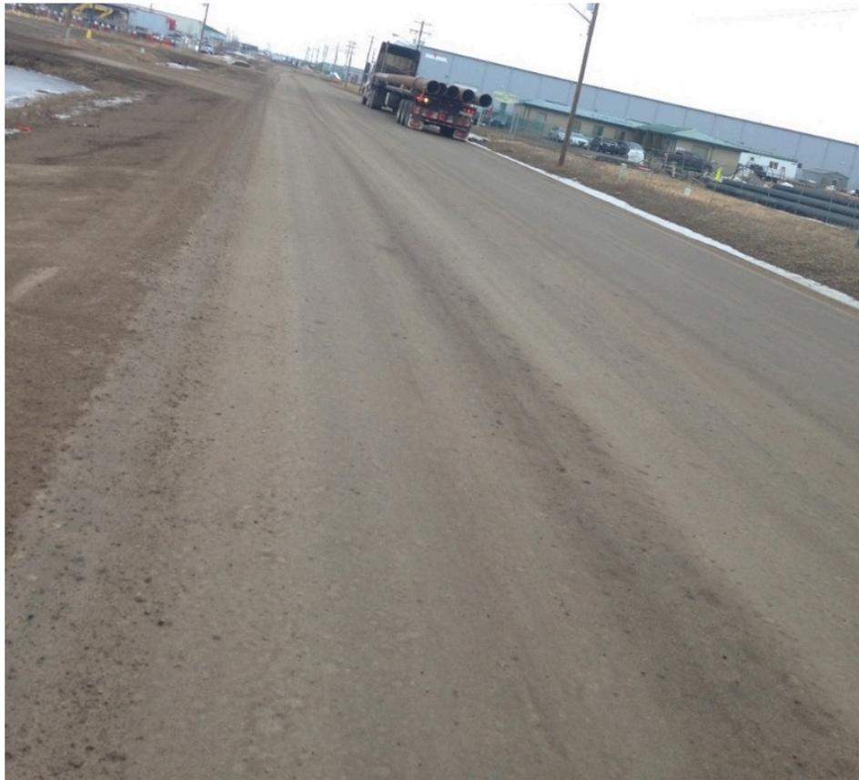
Figure 8: NPA Geocell-reinforced section in March 2015
