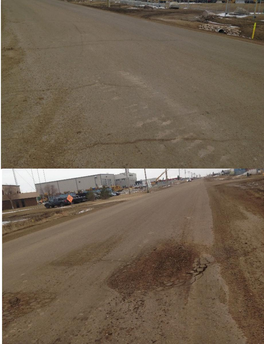
Figure 7: Pavement failures on CTB section in March 2015
