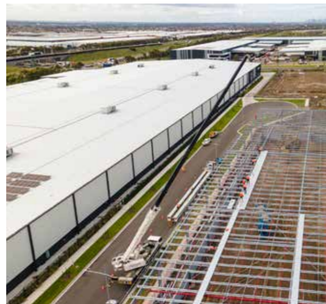
CRUSADER CARAVANS & INTEL ENGINEERING WAREHOUSE FACILITY
