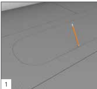
1 Draw ducts/grooves onto the wedi building board for installation of the heating system.
