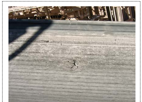
Impact damage is caused by large, sharp material striking the belt, resulting in a random nicking, scratching, or gouging of the top cover.
