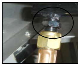
Gas Connection Leak Check
