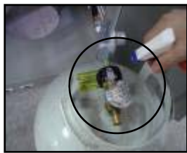
Gas Connection Leak Check
