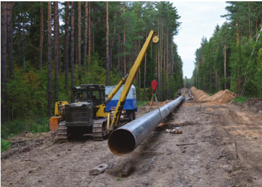
*A clear path. A pipeline or electrical transmission line generally follows a long, narrow stretch of land, called a right-of-way, which designates a safe and clear corridor to install and maintain the line.*
