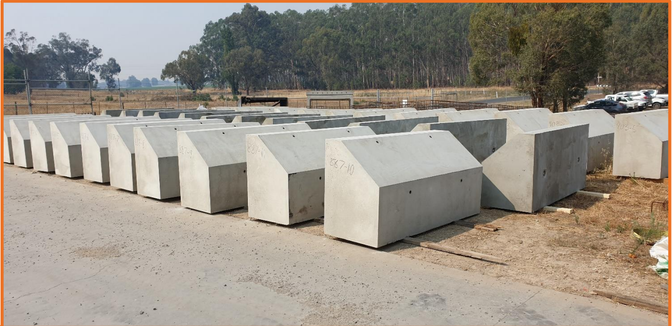
TBM Rolling Blocks ready for transport to site.
