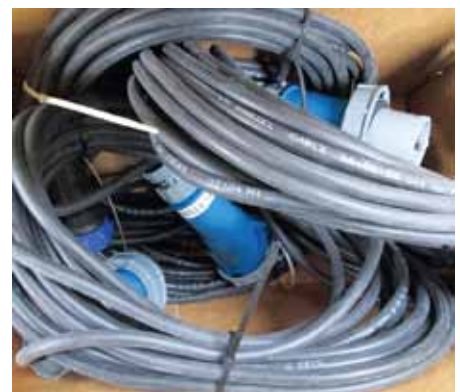
Electrical Power Cables
