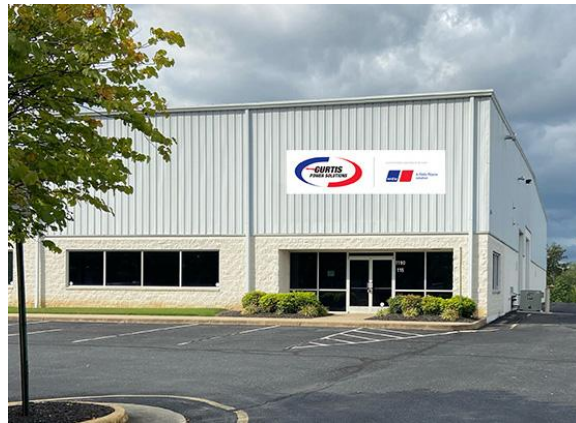
Curtis Power Solutions' new Fredericksburg location is in the heart of the I-95 Corridor.
