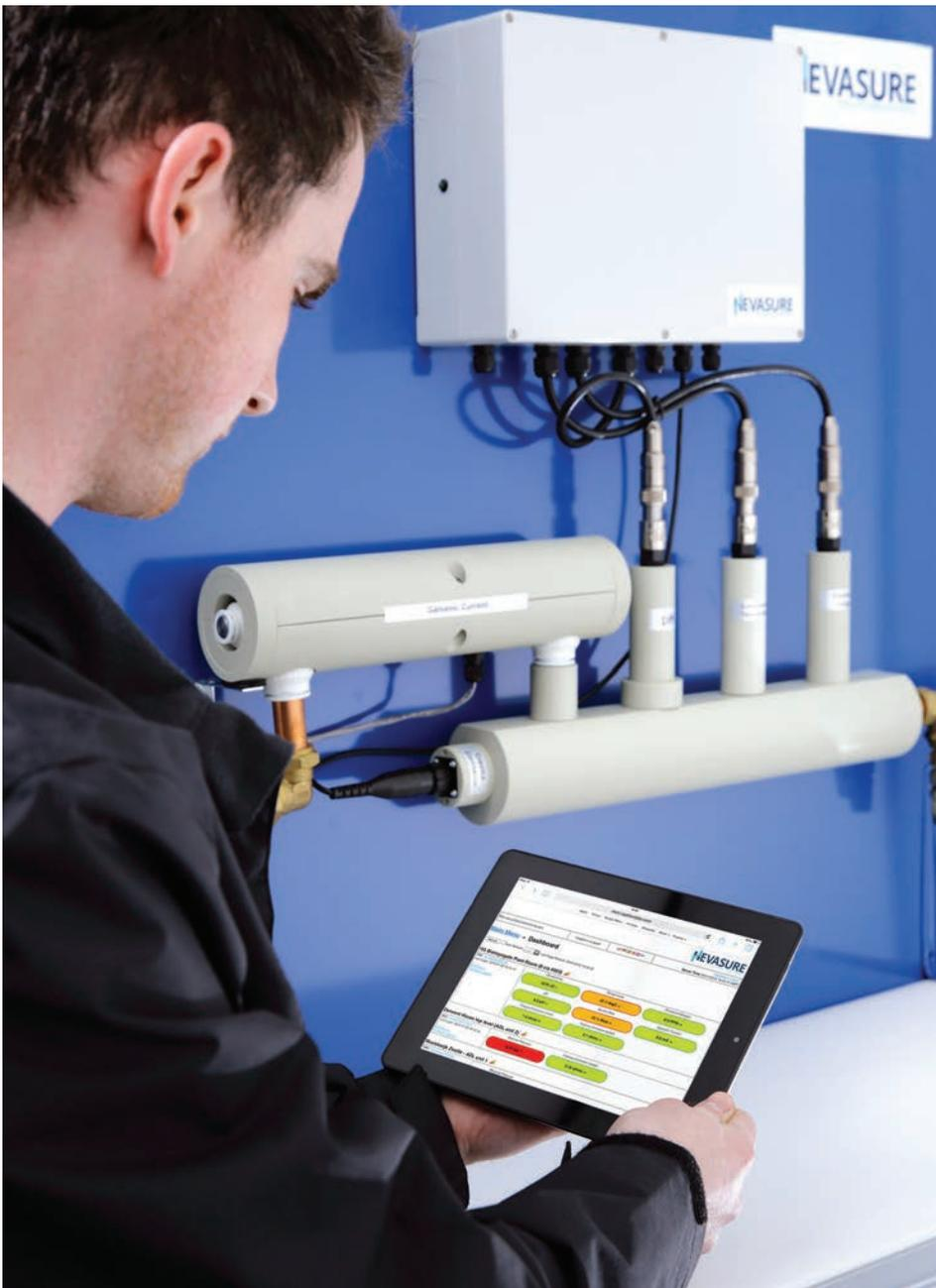
Our Hevasure monitoring system brought exclusively to you through WCS Group and Guardian Water Treatment, protects HVAC systems from corrosion damage by continuously and remotely monitoring the conditions that can cause corrosion BEFORE any damage occurs.
