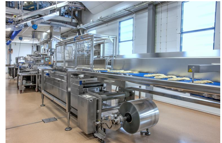
RE30 Thermoformer line installed at Arla Foods
