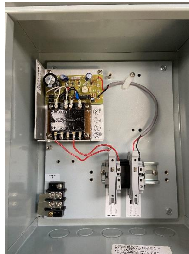
Legacy Power Cabinet (SPEEDCHECK-18)
