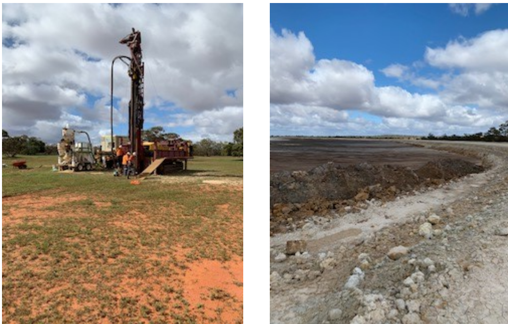
Exhibit 18 – Wonawinta – reserve drilling for silver oxide, fully compliant tailings storage with raised wall
