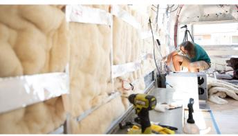
After the skins are put back up and you are drilling into the skins, be mindful of the drill bit catching the wool. Drill slowly and do not just pull the drill bit out. Rather, reverse it first, then remove it.
