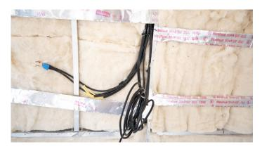
Tuck the wool behind wires. The wires will help hold it in place, and the wool will help to insulate the wires.
