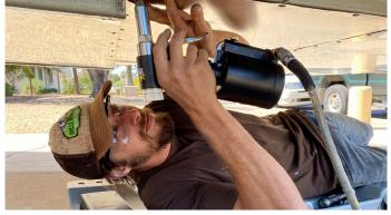
Rivet 3 sides of each piece of aluminum, then stuff the wool through the frame using a long pole or something like a broom to get it through the frame holes. Stuff in as much as you can fit. Then, rivet the final side of the aluminum.
