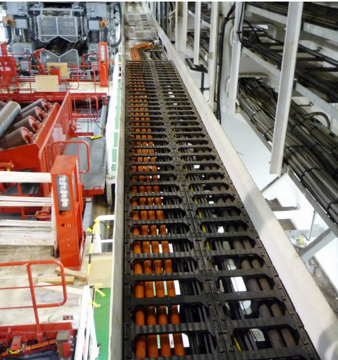
DNV-GL handling on pipe-laying ship Source: igus®
