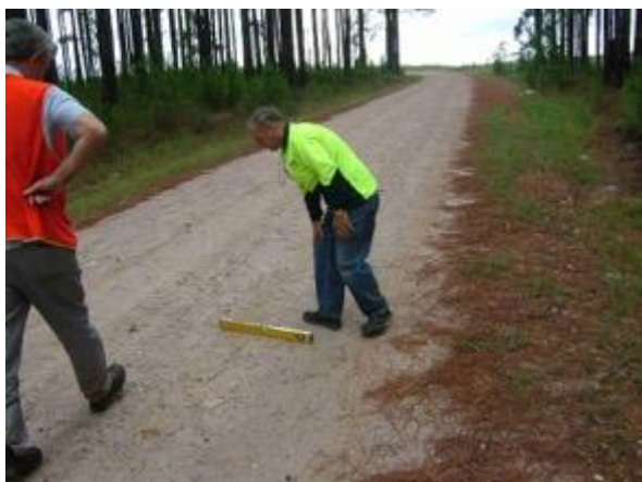
Figure C 34: Devices to measure actual road crossfalls
