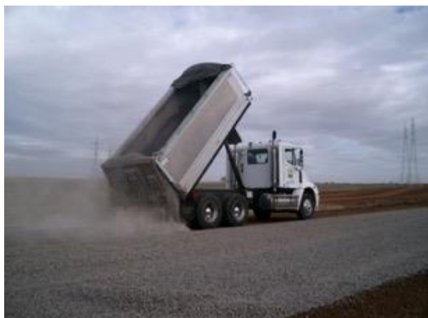
Figure 4.14: Tipping of pavement basecourse material
