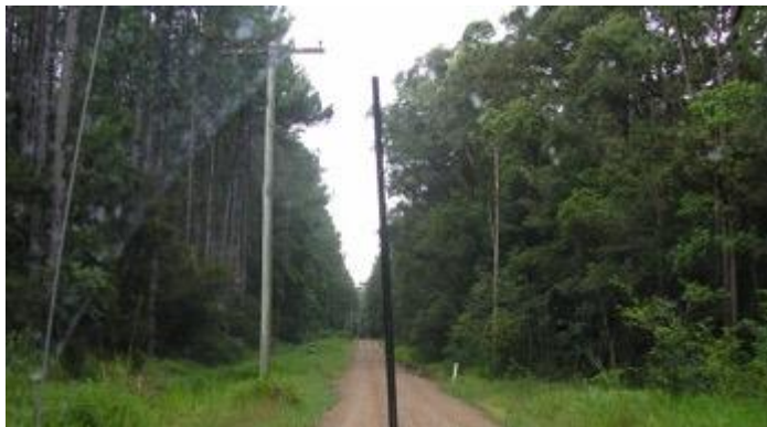
Hazards located close to the carriageway can have a major impact on the severity of a crash
