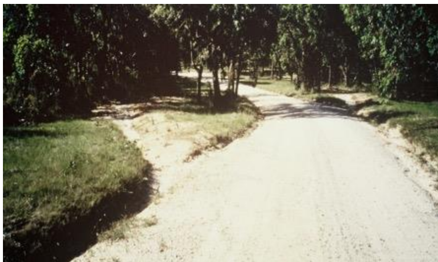
Figure C 41: Provision of a cut-off drain
