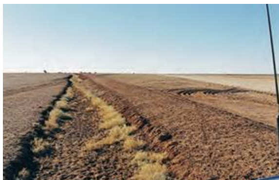
Figure A 14: A typical catch drain in an unstable arid environment
