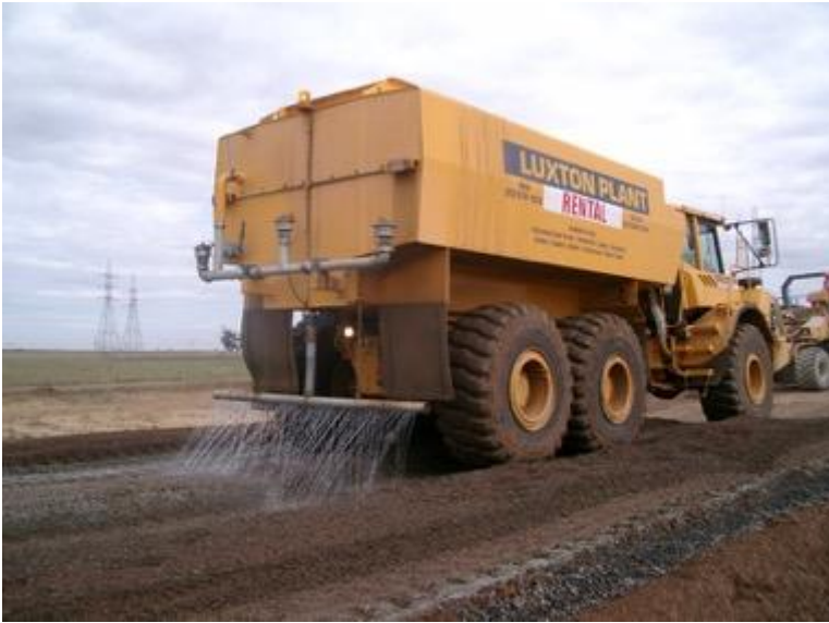
Figure 4.16: Water tanker with spray bar
