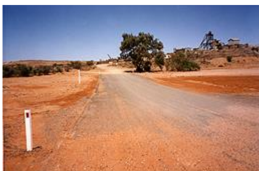
Sealed road to protect pavement surface
