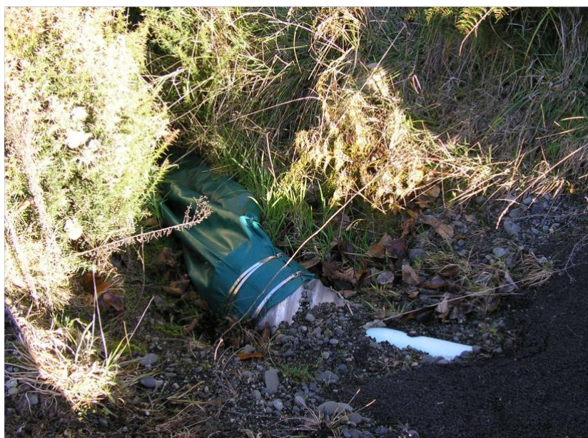
Figure A 12: Culvert sock
