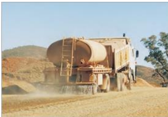
Figure A 32: Watering of road to reduce dust emissions
