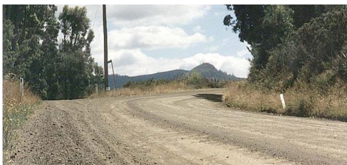
Drivers have restricted sight distance around this curve with no curve alignment markers or guide posts provided to delineate the tightness of the curve
