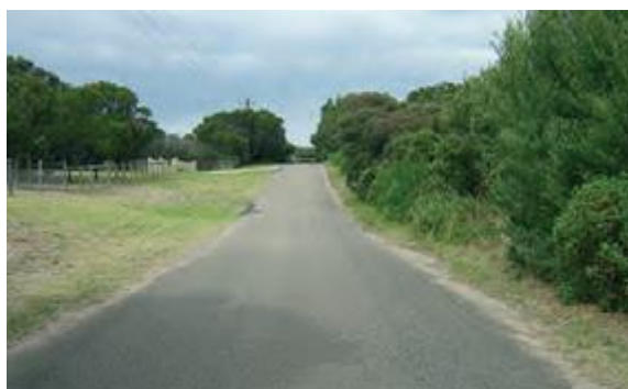
Paved road with a sealed surface
