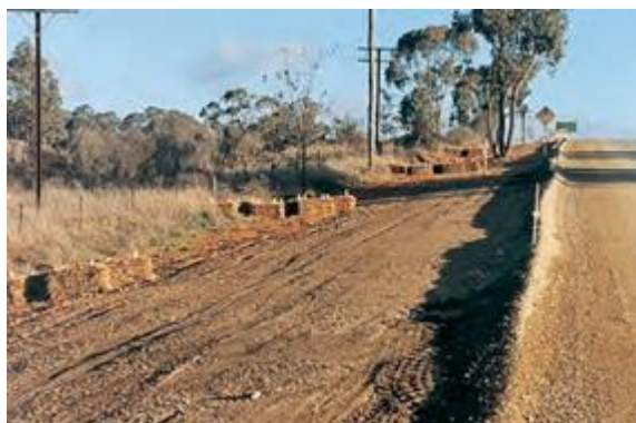
Figure A 26: Straw bales used as sediment traps
