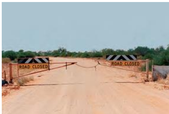
Figure 5.16: Typical barriers for road closure
