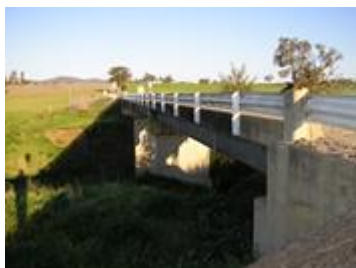
Concrete deck/steel beams
