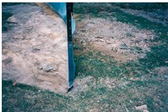
Figure A 24: Sediment fences are effective during road construction
