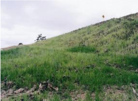
Figure A 22: Rapid reseeding of fill batter reduces potential for erosion
