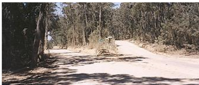
Figure C 22: An existing poor intersection layout with a low intersecting angle
