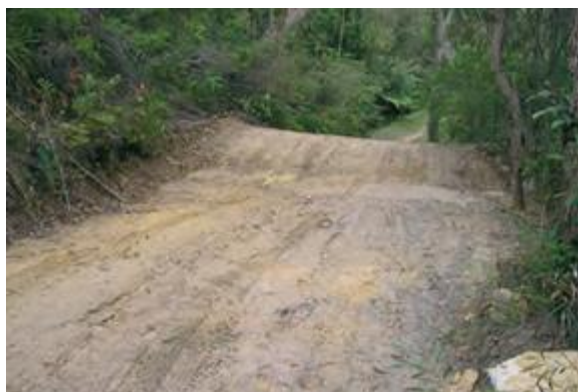
Figure D 17: Example of a rollover drain
