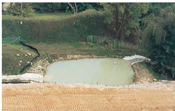
Figure A 27: Sediment basins intercept sediment laden run-off prior to release into waterways
