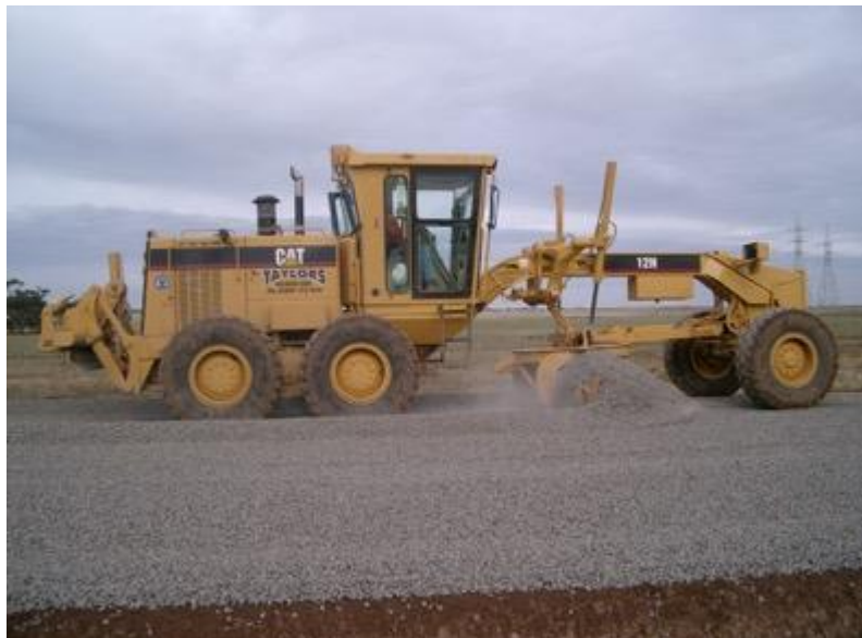
Figure 4.15: Grader spreading pavement material
