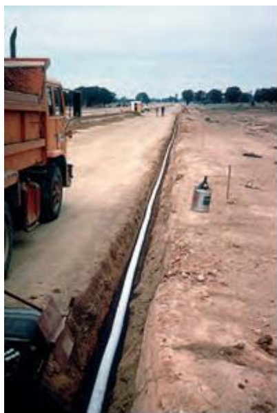
Figure 4.4: Strip subsoil drain installation
