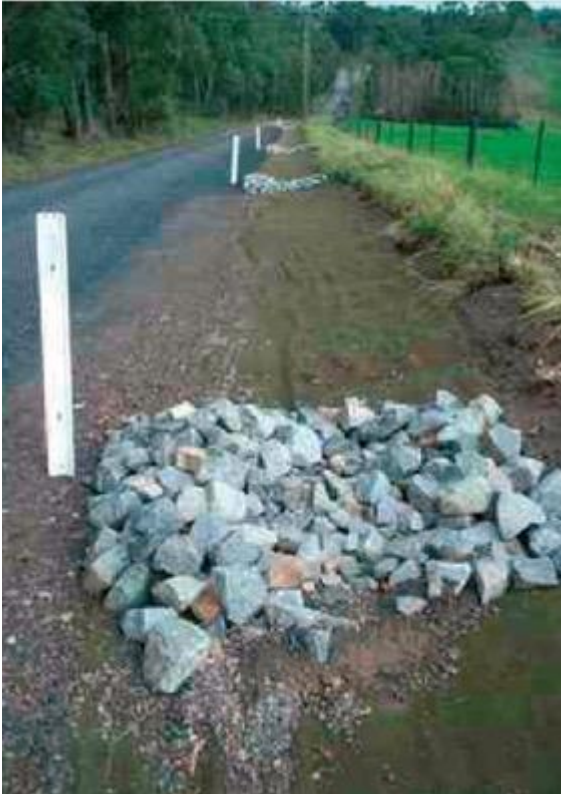
Figure A 8: Check dams in table drains
