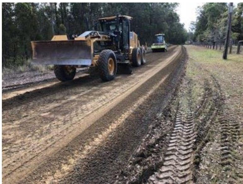
Figure 4.1: New road construction site
