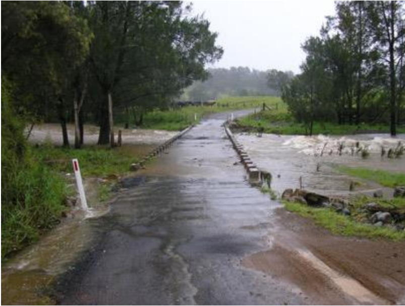
Figure C 56: Low-water bridge under heavy flows
