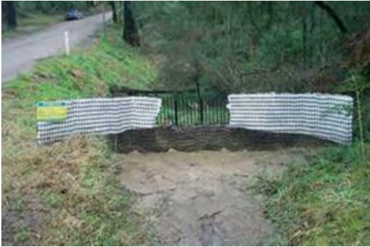
Figure A 36: Sediment filter preventing sediment from entering stream
