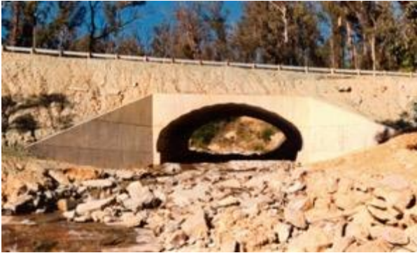
Figure A 16: Arch culvert maintaining natural river bed
