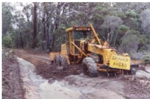
Figure E 9: Heavy grading
