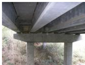
Prestressed concrete girders
