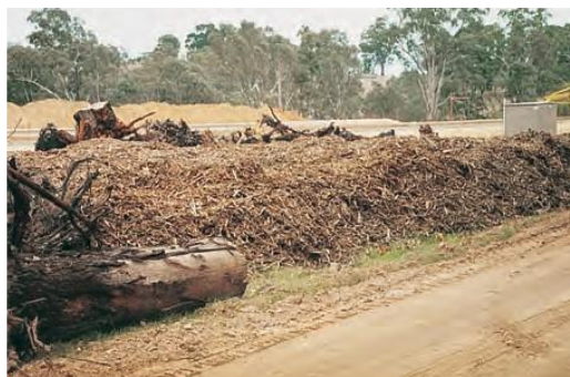
Figure A 20: Stockpiled mulch of a road construction site
