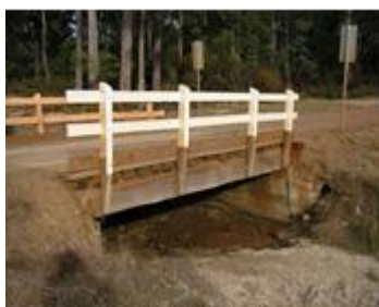
Single span timber bridge
