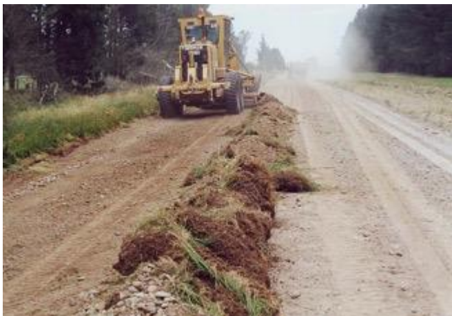
Figure 5.3: Light grading activities
