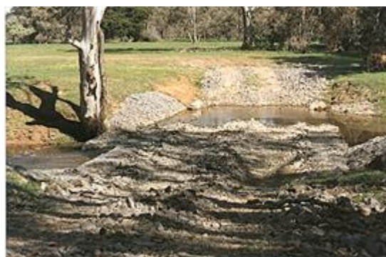
Use of rock gabions to strengthen road crossing
