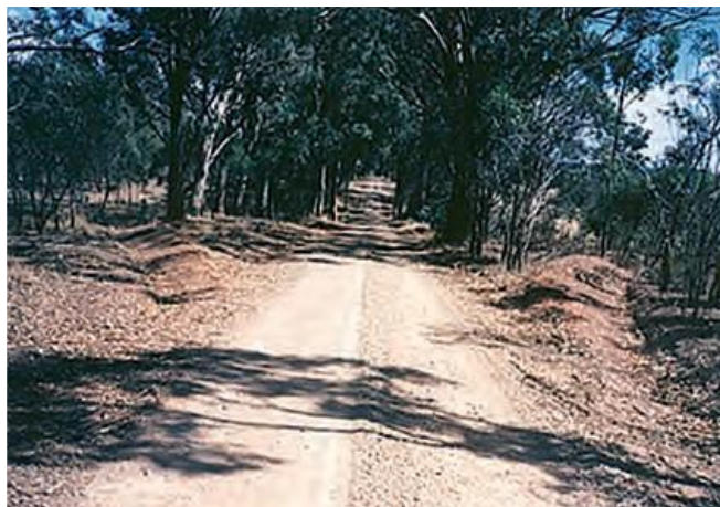
Figure A 6: Typical turn-out into a stable vegetation area
