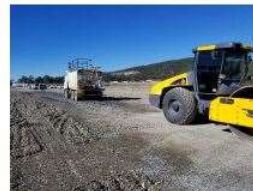
Moisture conditioning and roller compaction
