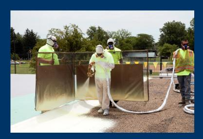
The chemicals, A (polyol/resin) & B (isocyanate), are pumped from separate containers through heated, highpressure hoses to an internal mixing spray gun.
