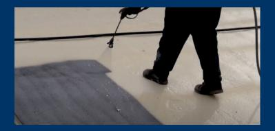
A thin application of silicone coating is applied over spray foam to protect the roof from UV rays.
