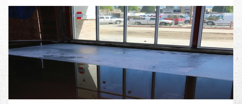
A properly installed curing blanket that retains moisture and remains flat on the slab helps keep CO<sup>2</sup> from reacting with the concrete surface, which minimizes efflorescence.
