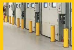
Bollards shielding door frames and shutter runners in a newly built warehousing and distribution center.
