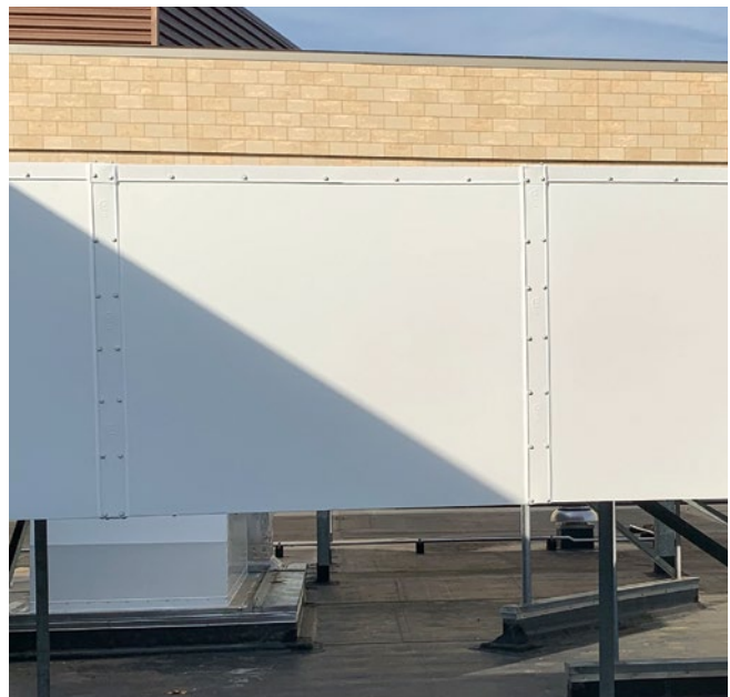
Interlocking panels help make the Techna-Duc® system virtually impervious to moisture and other contaminants.
