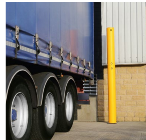
Higher level bollards give a strong visual alert for reversing HGV drivers, preventing costly damage to service yard infrastructure.
