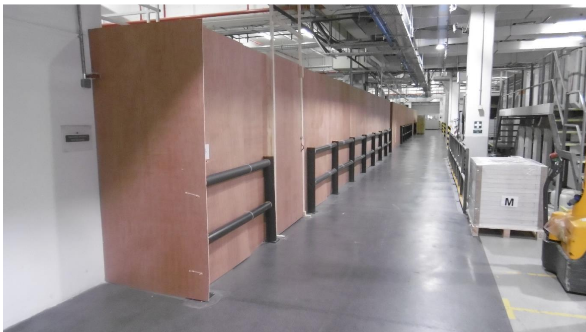
Figure 3. An example of a temporary wall to segregate an area of a factory and improve social distancing.
