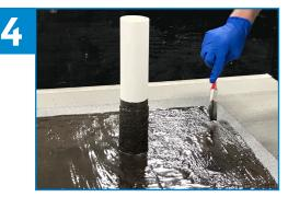
Once cured, apply a final coating of ALSAN Flashing at a rate of two gallons per 100 ft<sup>2</sup> to the pipe and field, extending approximately 1" past the previous coat.
