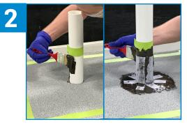
Apply ALSAN Flashing liberally with a brush at a rate of two gallons per 100 ft<sup>2</sup> to the pipe, wrap the fleece around pipe or penetration and coat with an additional layer of ALSAN Flashing.
