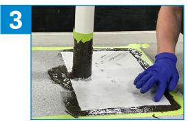
Apply ALSAN Flashing to the taped off field area at a rate of two gallons per 100 ft<sup>2</sup>, lay fleece into the first coat and apply second coating of ALSAN Flashing. Remove the tape.
