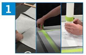
Pre-cut the ALSAN Flashing fleece to conform with SOPREMA published details, tape off the area using masking tape and dry fit fleece to ensure proper sizing.
