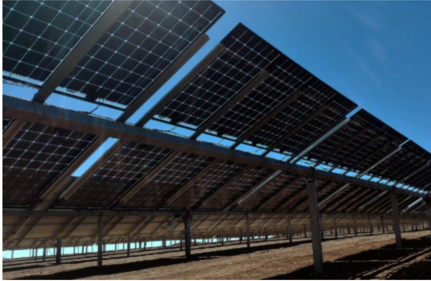
Figure 5.6: Picture of a 2V tracker using bifacial modules [27]
