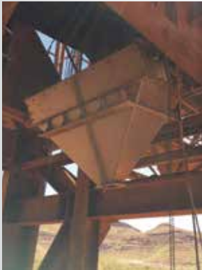
Washbox Being Installed
