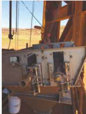
Washbox Being Installed
