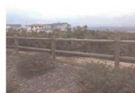
42" Post and Rail Drainage Basin Fence with Wire Mesh
