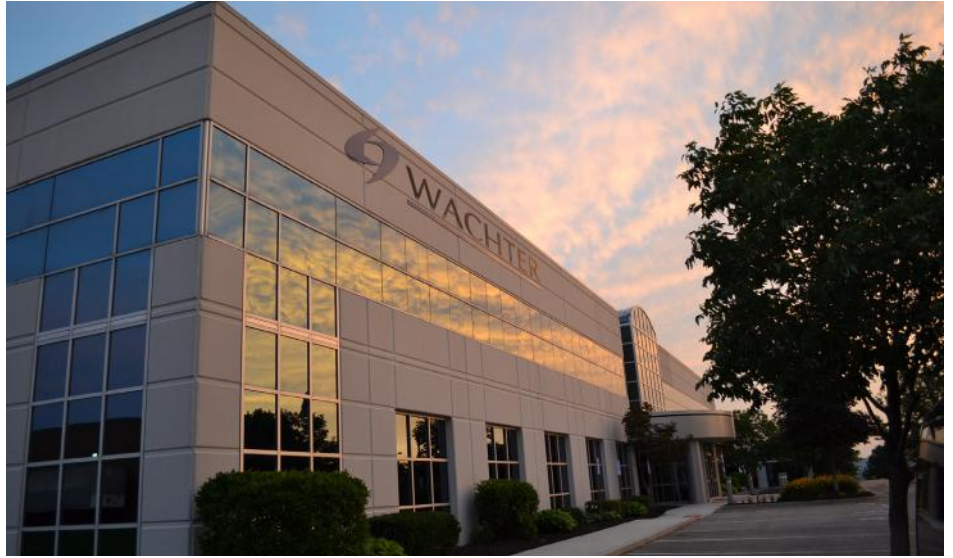
Wachter's corporate headquarters, located in Lenexa, KS
